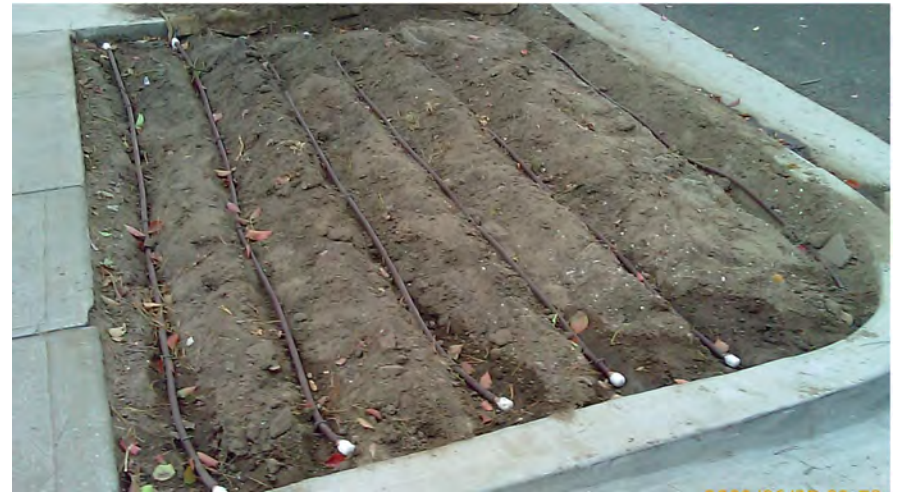
Fig A16 - Drip irrigation installation layout.
