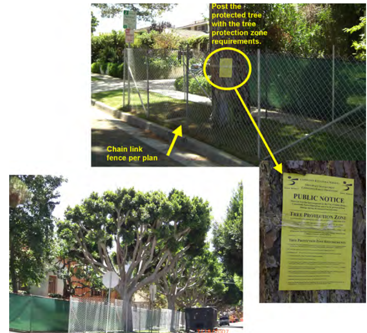
Fig A3 - Proper tree protection fence and notice.
