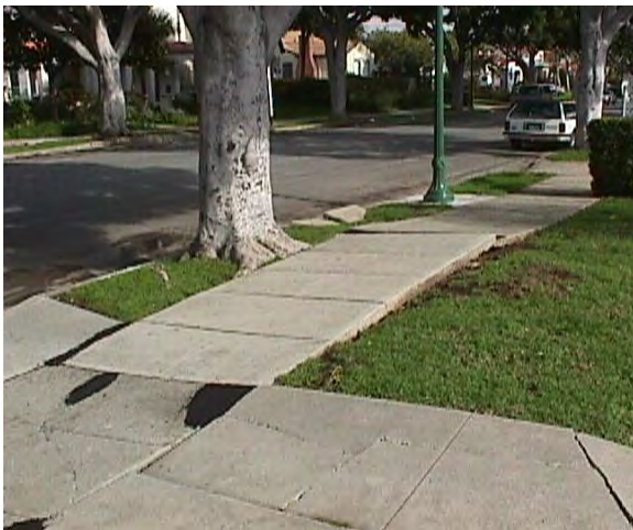
Displaced sidewalk and driveway surfaces. When trees are planted in growspaces that are too small, their root mass will eventually outgrow the space which results in hardscape damage.
