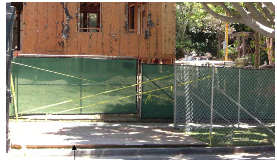
Steel plate for root protection
