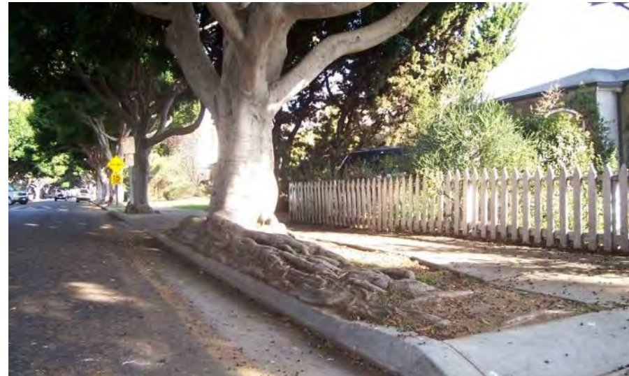
Fig A17 - Landscaping cannot be installed when tree roots take up the entire parkway.
