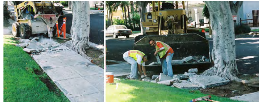
Fig A10 - Workers must take extra care when working in the critical root zones of trees and removing hardscapes such as sidewalks.
